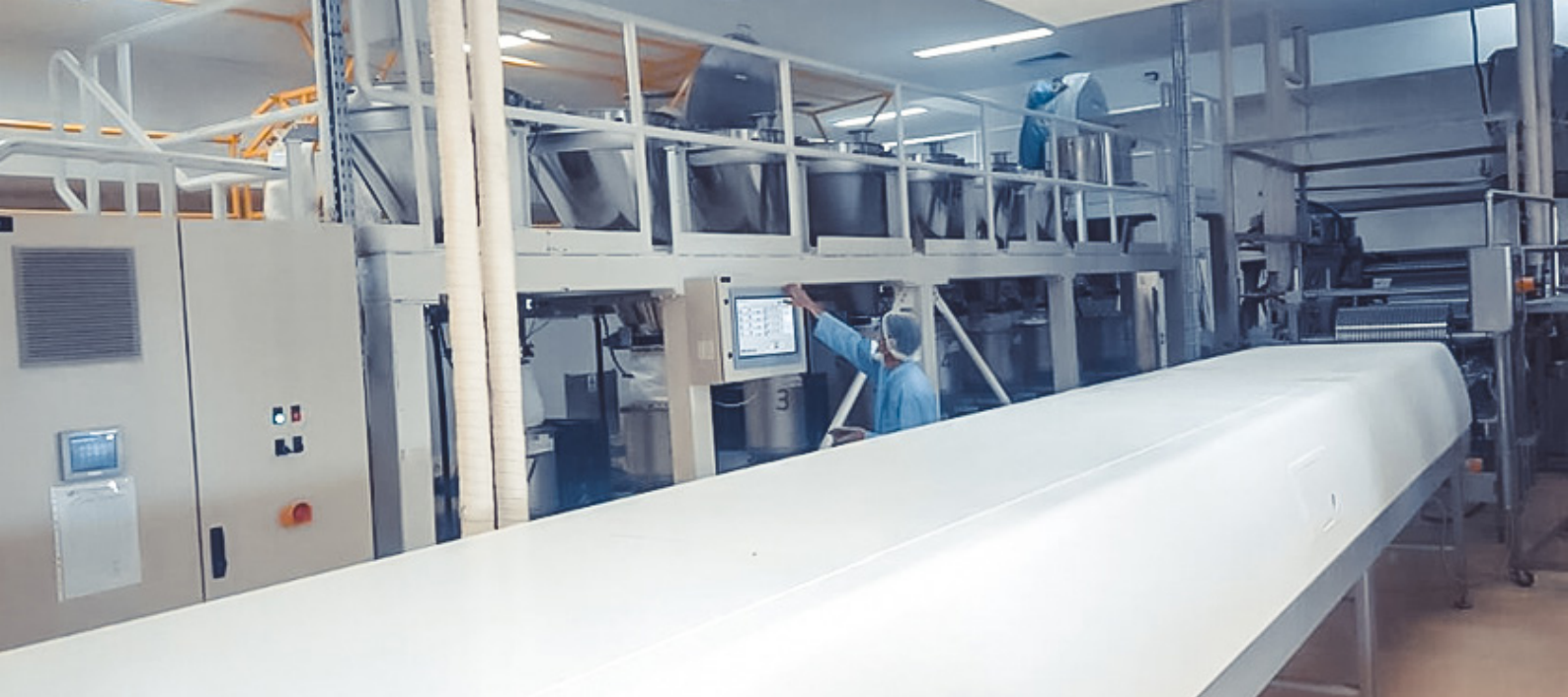
Continuous mixer for the binder and control panel with HMI screen
