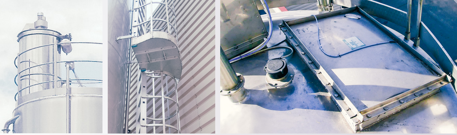
Powder recovering filters, ladder and bursting disk
