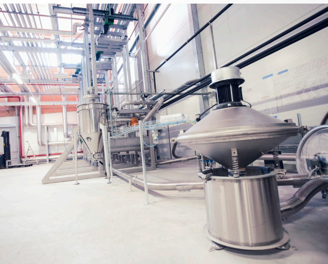
Left to right, top to bottom: chain hoist to lift the bags; antidust filter; sifting system; multiline feeding
