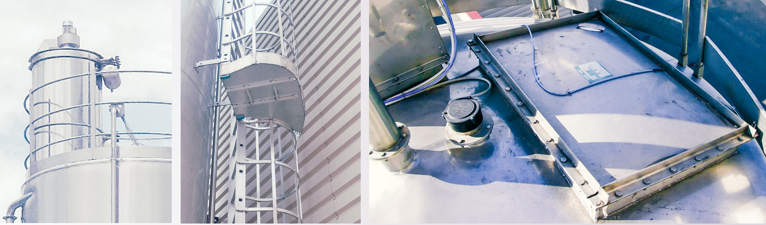
Powder recovering filters, ladder and bursting disk
