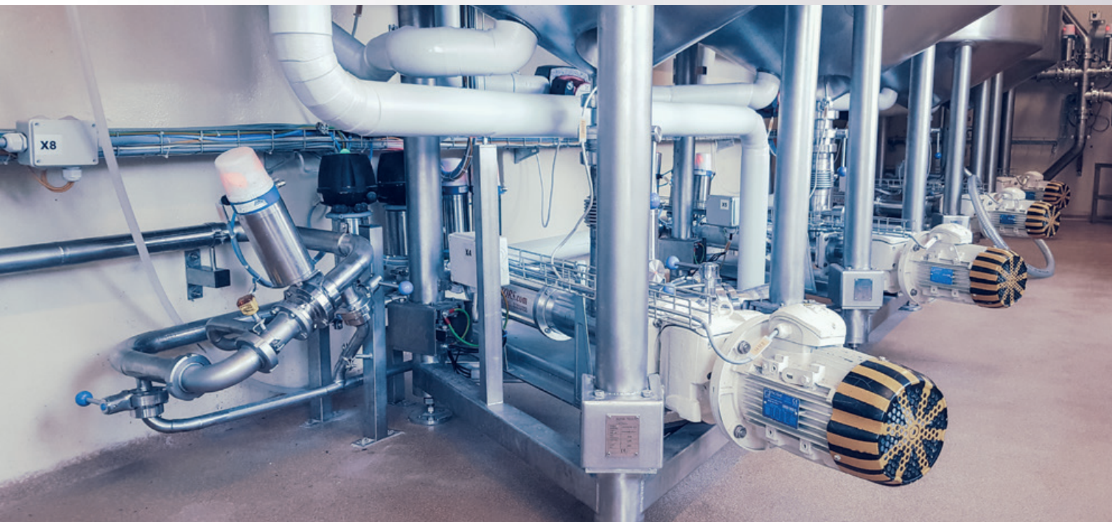
Sourdough preparation group for medium production volumes. Above: detail of stirrer and inspection hatch. Below: dosing system with total emptying
