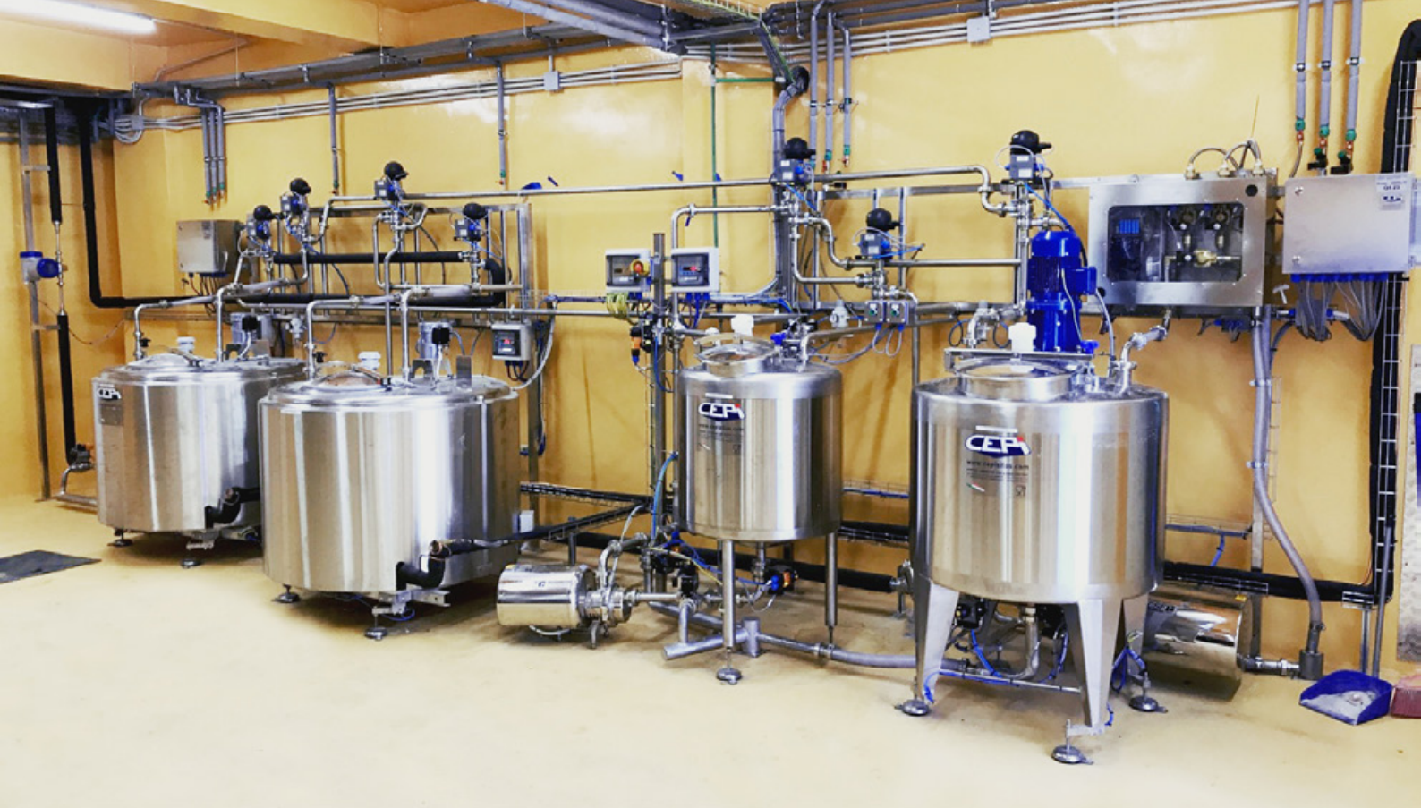
Clean In Place system for yeast line
